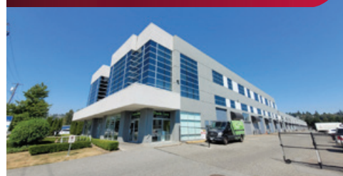
#13 & 28 - 145 Schoolhouse St, Coquitlam
